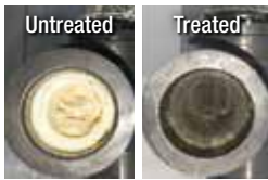
Water heater outlet
